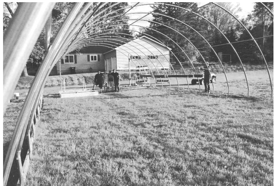
Students Cody Brown, Luke Seaney, Kevin Eggers and Jake Neuman take a break from framing raised beds to pose for the camera.
